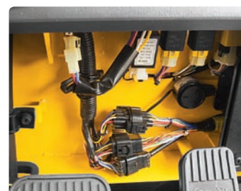
Easy access of electrical Components Various electric parts are centralized in dash board resulting in improvement in maintenance.
